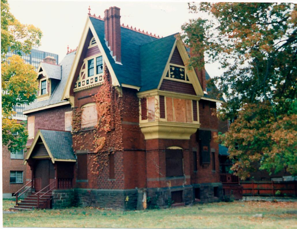
This building is presently vacant and represents one of the original estates in Asylum Hill and careful restoration is recommended. There is some structural damage due to settling of the foundation. Preliminary estimates are \$125,000 to remedy just the structural problem. The AHRZ with the help of the Antiquarina Landmark Society is looking for an individual or corporation who is willing to take on this project. The AHRZ considers this a top priority.
