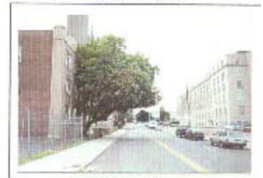
Lack of activity after 5 p.m.
