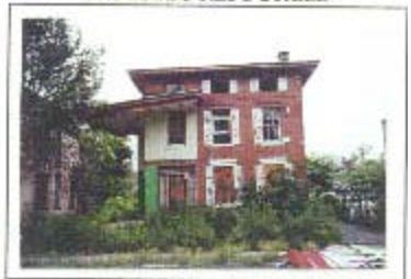
Vacant buildings need protection from the elements and vandalism
