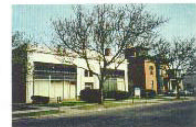
The wide variety of building types allows for a range of uses
