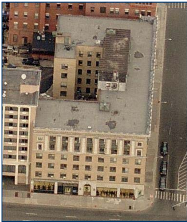
410 Asylum Street is being converted into apartments
