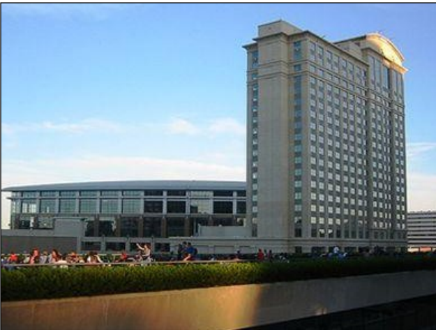
The Marriott Hotel at Adriaen's Landing
