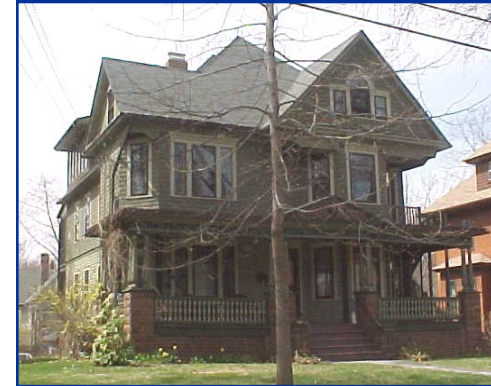
Neo-Classical Revival– Kenyon Street
