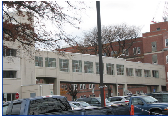
St Francis Hospital Expansion
