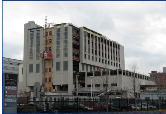
St Francis Hospital Surgical Tower
