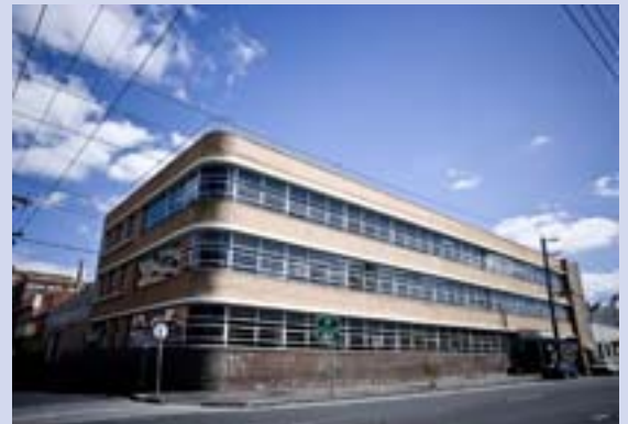
Collingswood NJC, Collingswood, Australia
